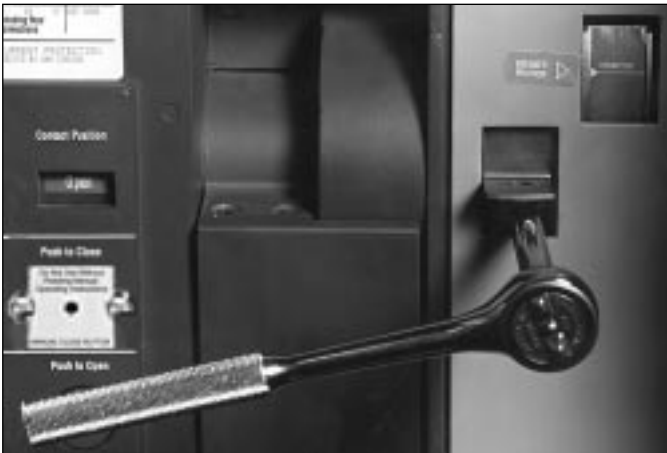
Figure 6-1 Drawout with Socket Wrench
