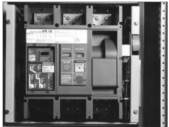
Figure 3-2 Insulated Case Circuit Breaker
